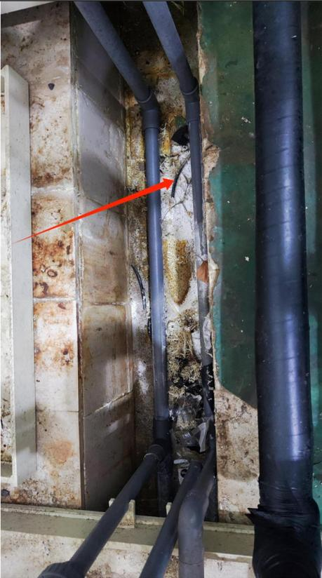
A photograph showing a drainage ditch in an industrial setting. The ditch is lined with concrete tiles. One tile is missing or severely damaged, revealing a dark, possibly liquid-filled area underneath. A red arrow points to this damaged area. Several black pipes run vertically along the ditch. |
